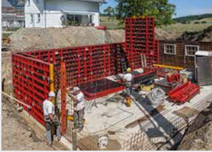
Wall Formwork
