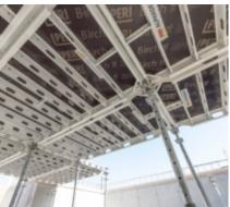
**High level of productivity**The large powder-coated aluminium panels are particularly efficient for projects with large spans.
